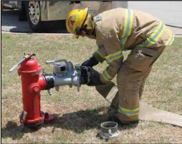
**Step 2:** Connect LDH and a 2½-inch (65 mm) gate valve to the hydrant. Lay hose to street, folding approx 3 feet (1 m) back onto itself (place two full counterclockwise twists in the hose if sexless couplings are not used).
