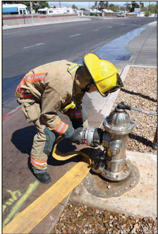
**Step 2:** Connect LDH to hydrant and lay hose to street, folding approx 3 feet (1 m) back onto itself (place two full counterclockwise twists in the hose if sexless couplings are not used).
