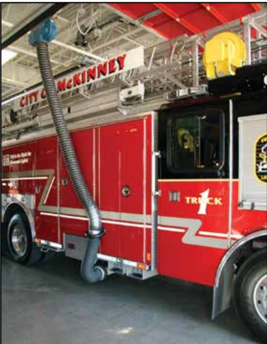
**Figure 10.5** Apparatus exhaust capture systems reduce air pollution in apparatus bays.
