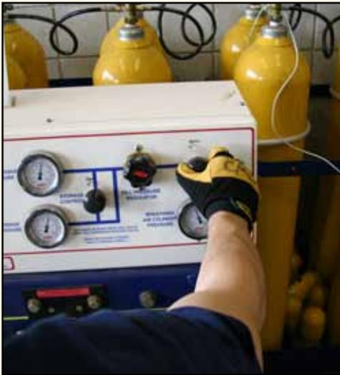
**Step 8:** Open the manifold valve (if applicable), and again check the fill pressure.
